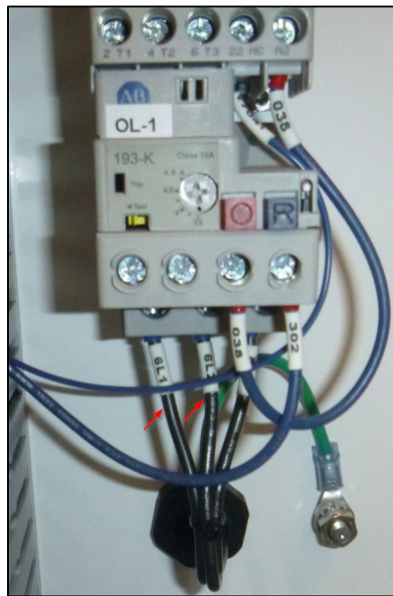
Figure 3: Incoming Power Legs Swapped Example
