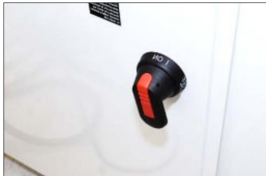
Figure 2: Power Switch "On"
